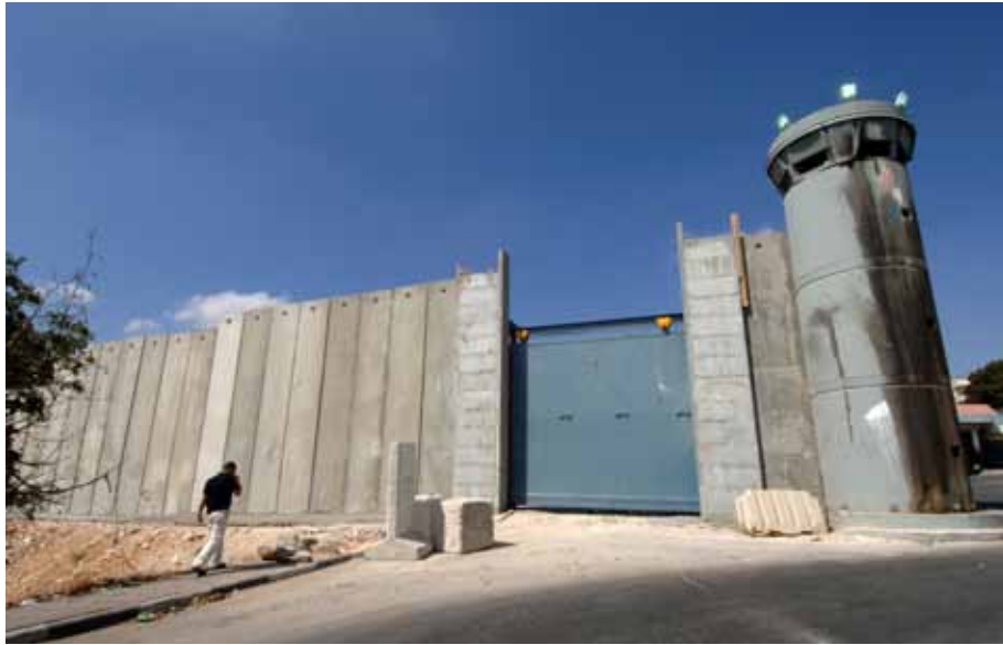
The Israel separation barrier restricts economic opportunities for many people in the West Bank. David Snyder for CRS
